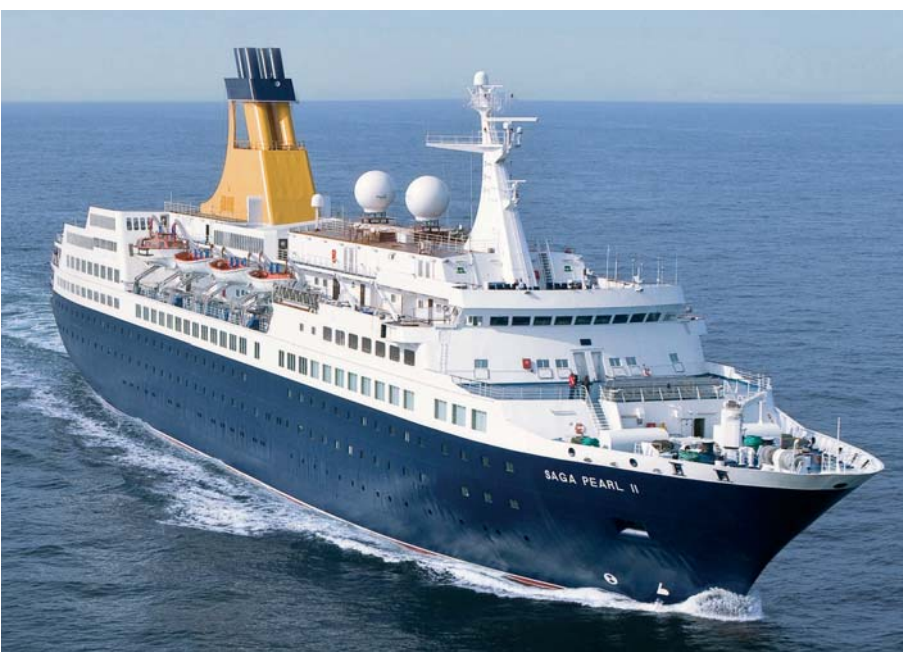
After outstanding results with existing vessels Ecospeed was chosen as part of a cruise vessel's complete refit
