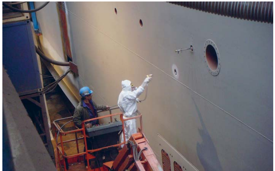
Application of Ecospeed on newbuild cruise vessel
