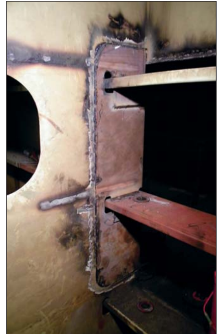
New frames after installation
