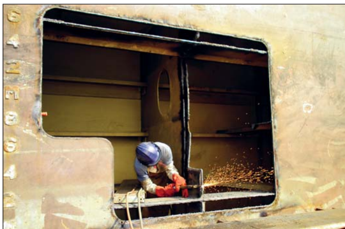
Preparing the edges of frames prior to installation of new ones
