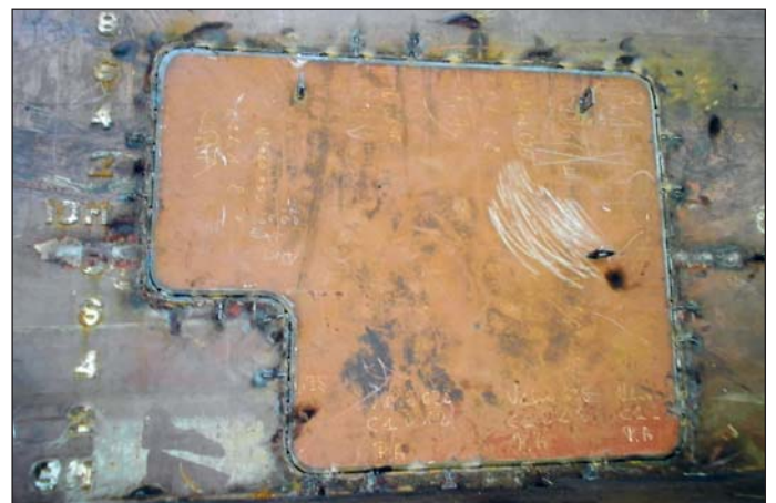
New insert prior to full penetration weld
