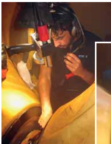
Right: The Hydrex flexible mobdock allows The company to create a dry underwater environment.
