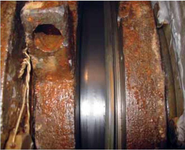
Damaged stern tube seal.
