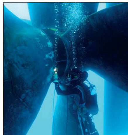
By performing repair and maintenance work underwater, hire time is minimised.
